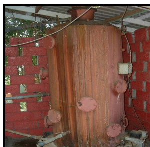
Audits found many examples of improper insulation: (B): Hot water boiler, lacking insulation and hole in roof (BL): Un-insulated attic above conditioned guest suites. (L): Damaged/missing insulation on refrigerant piping
